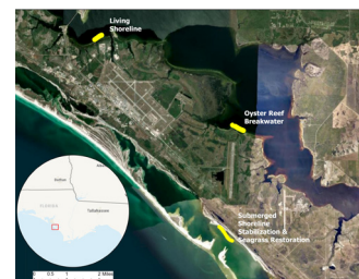
NBSs currently in the planning and design phase for TAFB include the Living Shoreline, Oyster Reef Breakwater, and Submerged Shoreline Stabilization & Seagrass Restoration projects.
