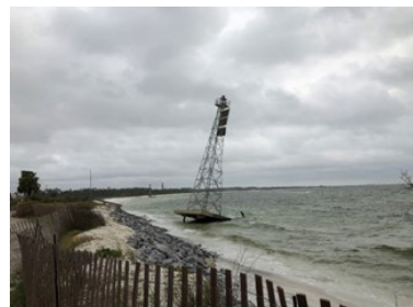
Shoreline damage along NAS Pensacola following a storm. Credit: Escambia County NRM.
